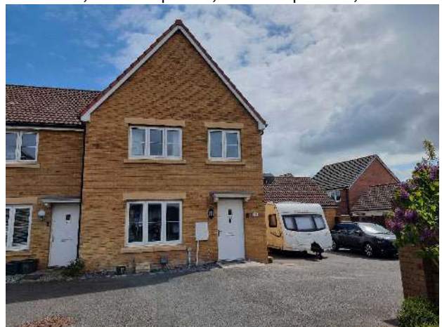
BS23 3HB, 83 Mendip Road, WestonsuperMare, BS23 3HB
