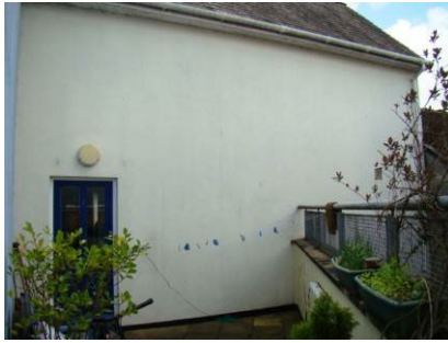
Burns Court, Broad Street, Modbury, Ivybridge
