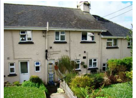
Beacon View, Bittaford, Ivybridge
