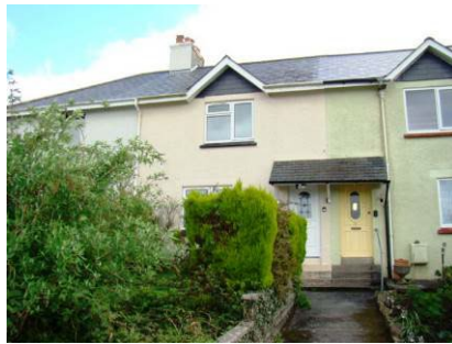
Beacon View, Bittaford, Ivybridge
