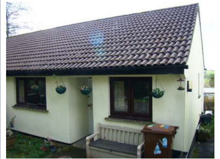
Beacon View, Bittaford, Ivybridge
