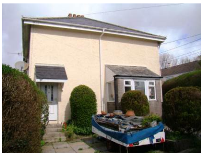
Beacon View, Bittaford, Ivybridge
