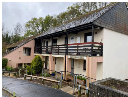
Bowingsleigh PLmontagu Road, Kingsbridge
