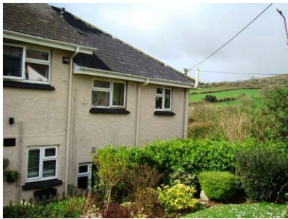
Beacon View, Bittaford, Ivybridge
