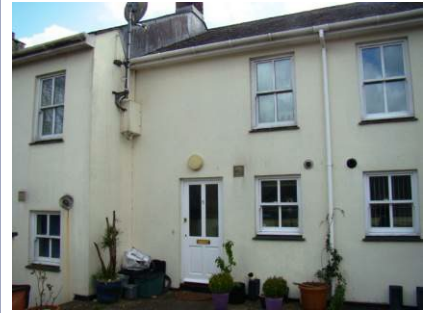
Burns Court, Broad Street, Modbury, Ivybridge
